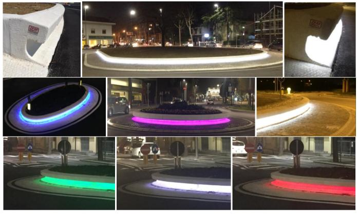
The roundabout has a new patented indirect LED lighting system. Thanks to the use of LEDs, the system's consumption is highly efficient and is practically maintenance-free.
