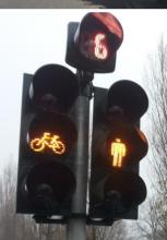
The LED technology used in **Traffic Light Systems**, unlike traditional lanterns with incandescent lamp optics, is more reliable, considerably reduces management costs given its lower current absorption, needs no maintenance at all and avoids false signalling caused by sunlight (the Phantom effect).
